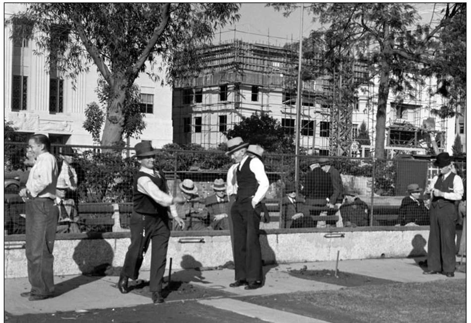
Several men, most wearing hats, can be seen pitching horseshoes at the public horseshoe court in Lincoln Park, Long Beach. Several others sit on long benches behind the fence. Across the street, in the background, a building is surrounded by scaffolding. WPA Collection.
